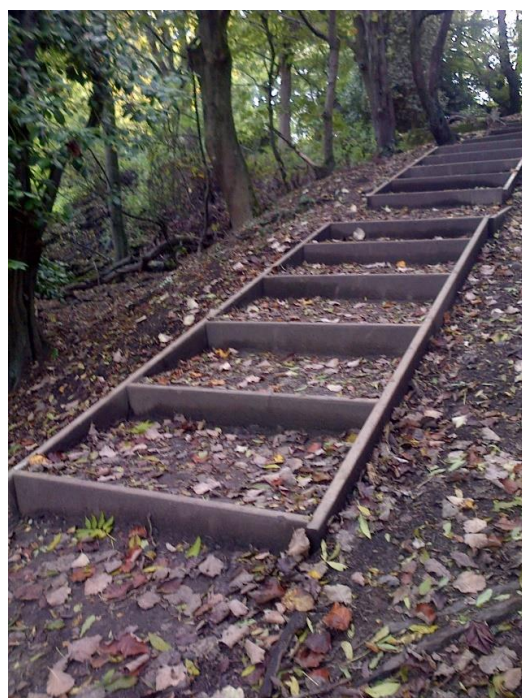
New steps in Beamont Park
